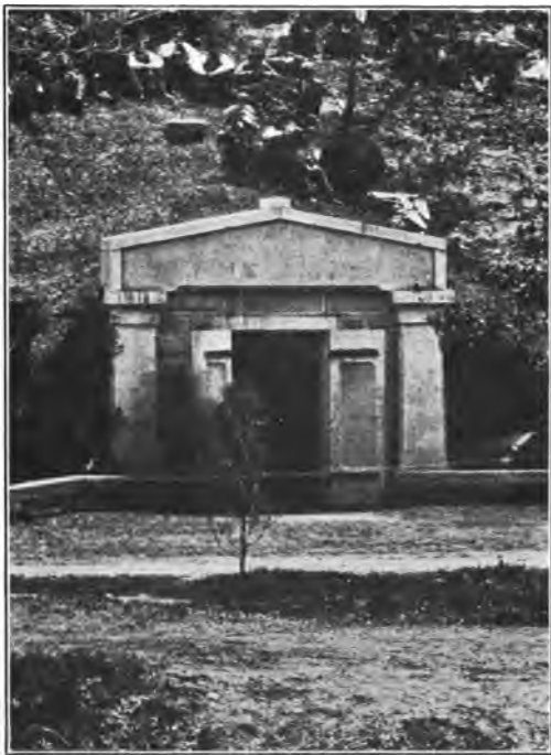
FACADE OF PUBLIC VAULT Oak Ridge Cemetery, Springfield, Illinois, in which the body of Lincoln was placed, May 4, 1865
